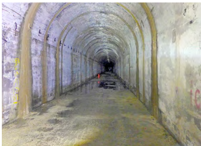
Concrete lining in the central tunnel (B). All in excellent condition
